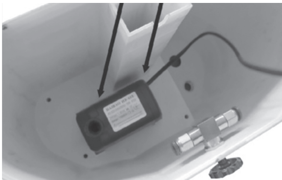
6. Put the submersible pump in the tank.
